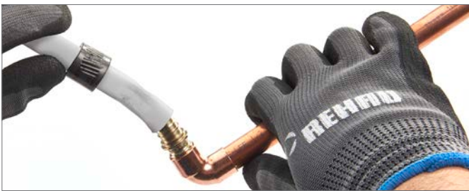
Fig. 5.10: Removing pipe from LF brass fitting
