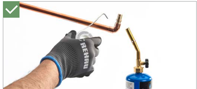
Fig. 7.22: Solder prior to making EVERLOC+ connection
