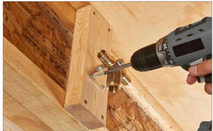
Fig. 7.1: Mounting FIREPEX sprinkler fitting
