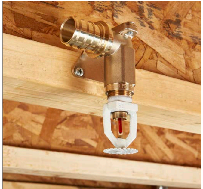
Fig. 7.7: Recessed pendant sprinkler mounting example
