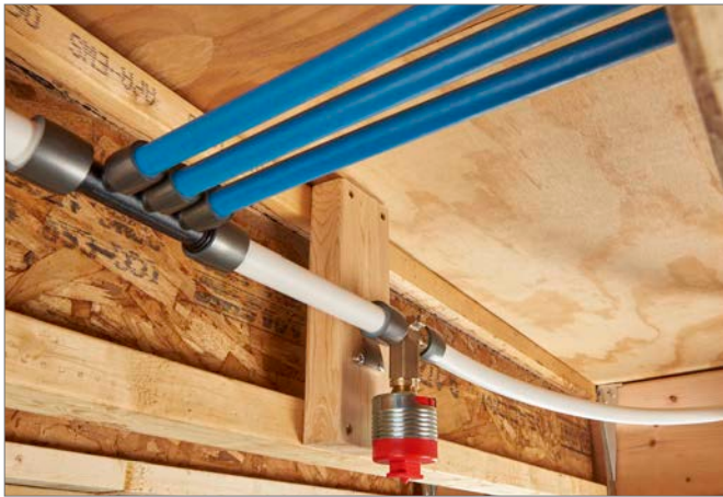
Fig. 6.2: Domestic cold water plumbing connection
