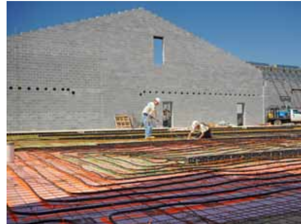
Watts Water Technologies provided 32,000 linear ft. of 3/4-in. Watts Onix synthetic rubber tubing for the West Friendship Fire Department in Howard, Md. Eliminating the potential for costly slips and falls are a key reason for installing snow-melt systems.
